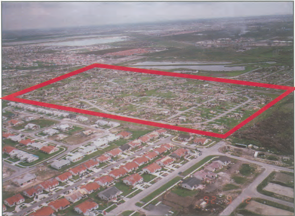
FIGURE 21. Aerial photo of damage area. Shows building performance difference between manufactured homes (outlined in center) and conventional residential buildings (lower left).
